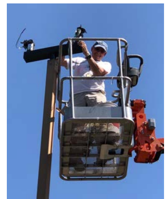
Figure 8 - Threading Wire through Fixture Mounting Brackets
