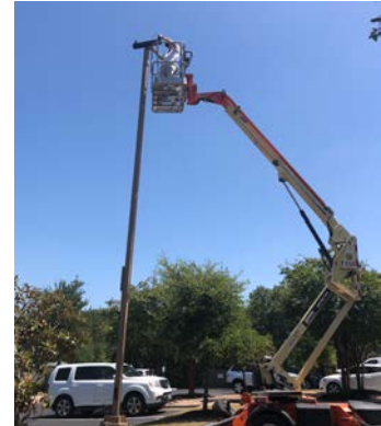
Figure 7 - Installing of Bullhorn
